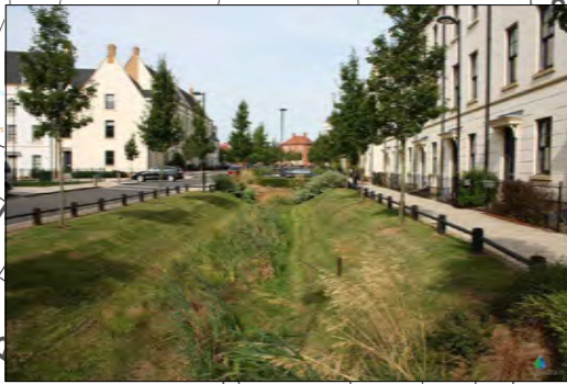
Insets between the North and South parcels of the site can be used to drain excess flow, whilst utilising the green bund beneath the overhead cables
